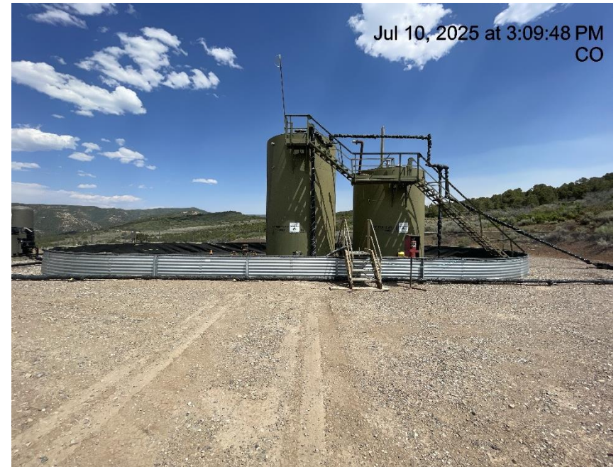
Photo # 1426 Tank battery lacks required signage
