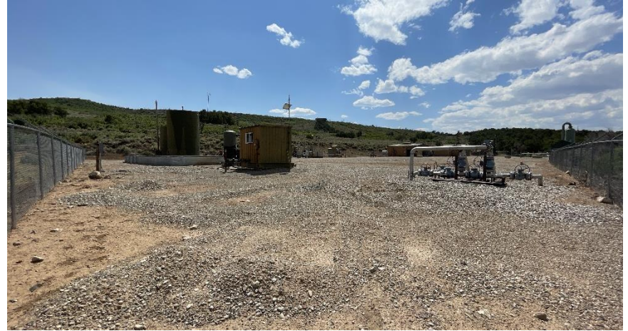
North East corner of location.
