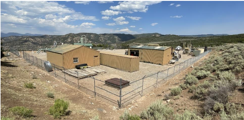
South West corner of location.
