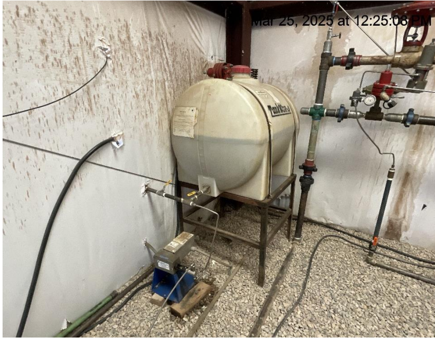
Photo # 7148 From inspection/audit 708906125 conducted on 03/25/2025 Chemical tank in compressor building lacks BMP's
