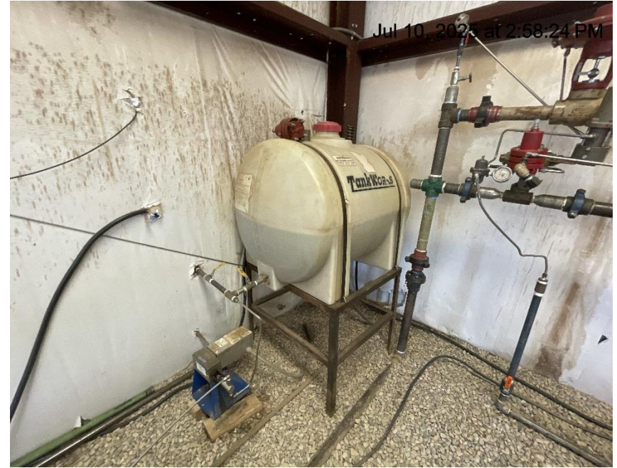
Photo # 1427 Chemical tank in compressor building lacks BMP's
