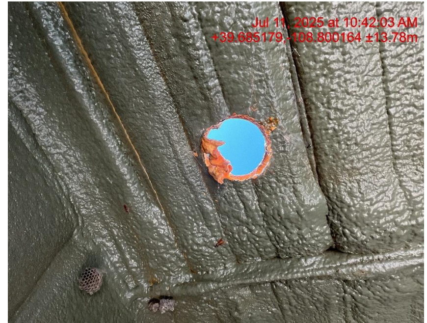
Photo # 9631 Hole in meter house open to wildlife/available for entry by wildlife
