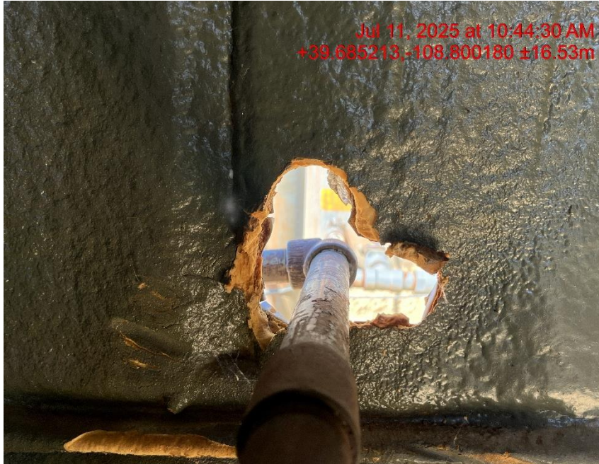
Photo # 9634 Hole in meter house open to wildlife/available for entry by wildlife
