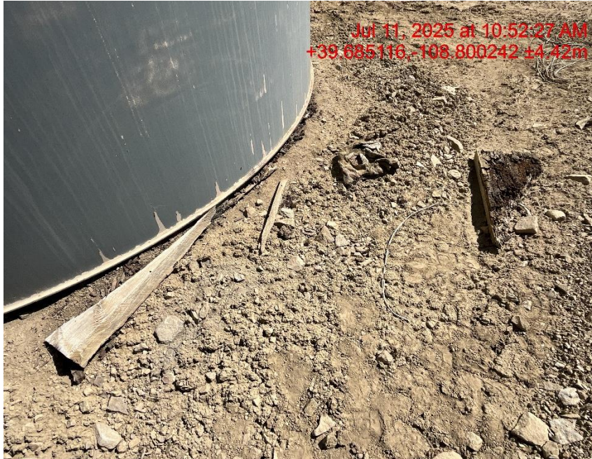
Photo # 9638 Debris on location
