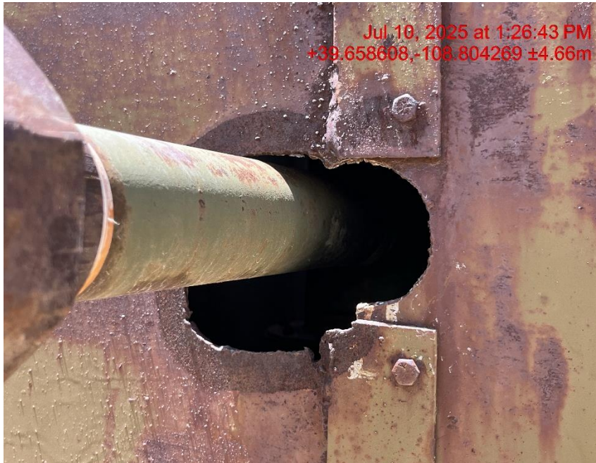
Photo # 9545 Hole in separator building open to wildlife/available for entry by wildlife
