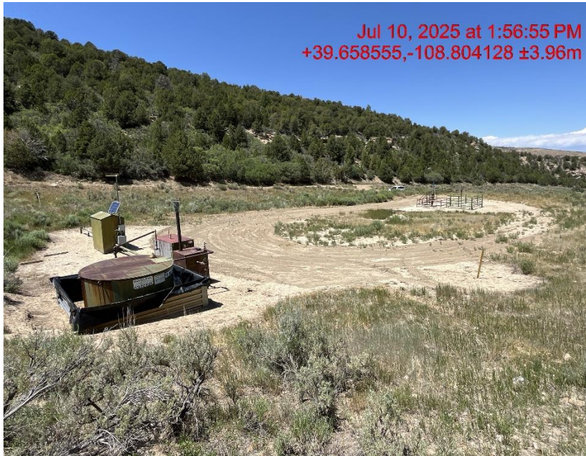
Photo # 9568 SE corner of location
