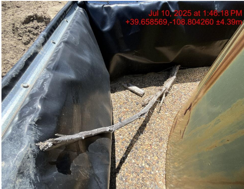
Photo # 9563 Debris on location
