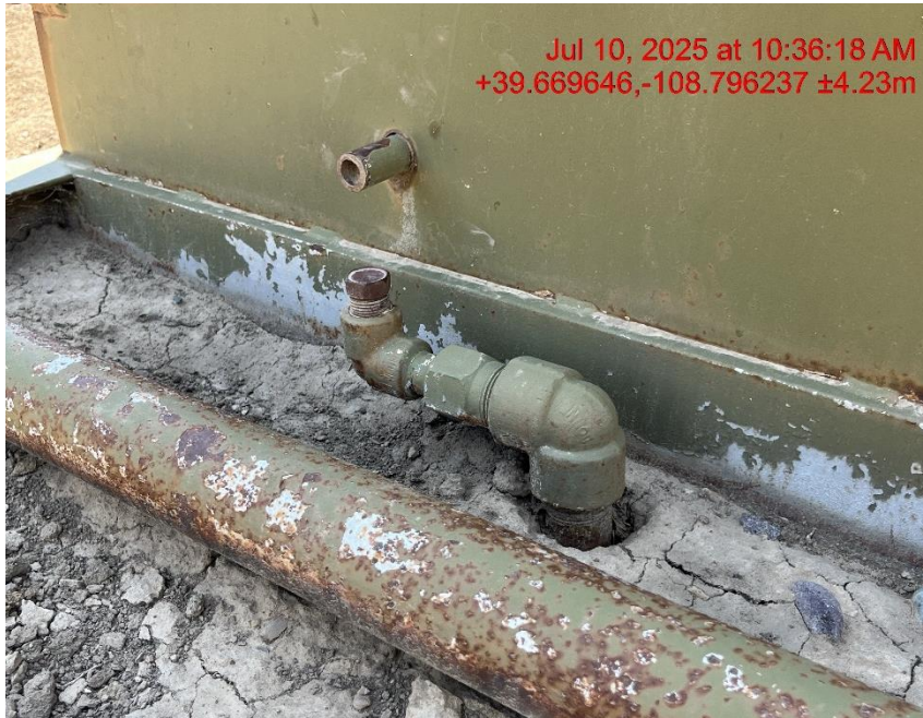
Photo # 9446 Unused flowline does not comply with CECMC 600 & 1100 series rules
