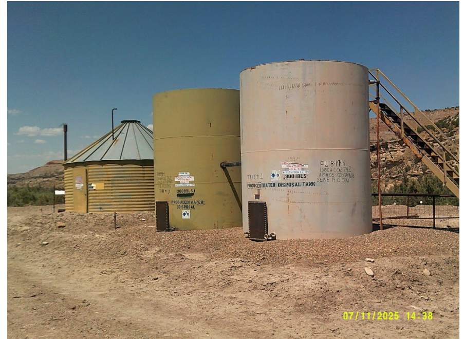
Tank battery and Pump housing
