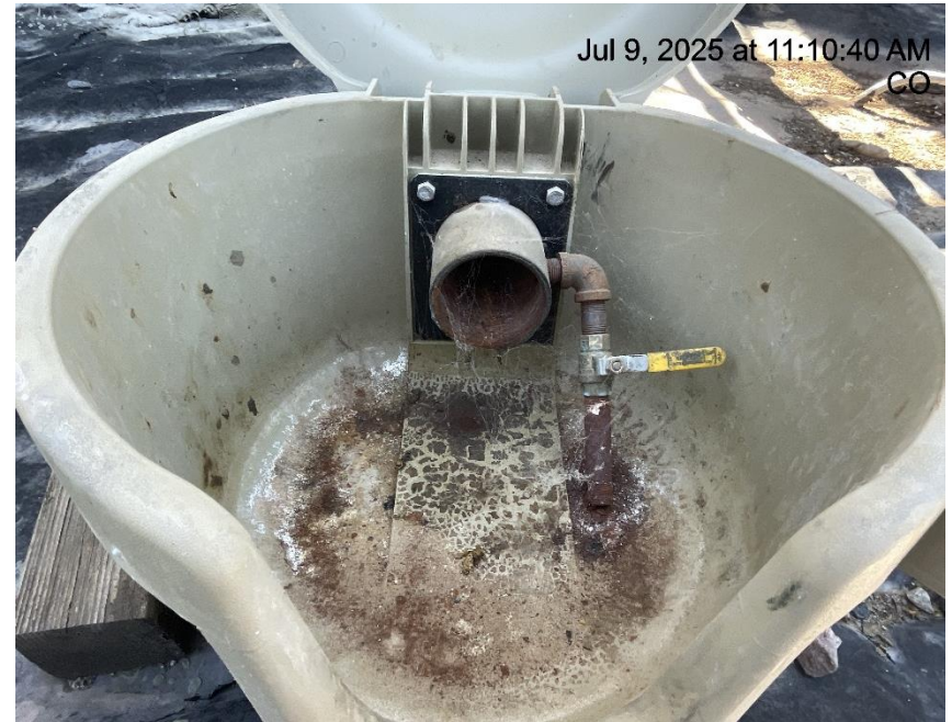
Photo # 95 Open ended load line
