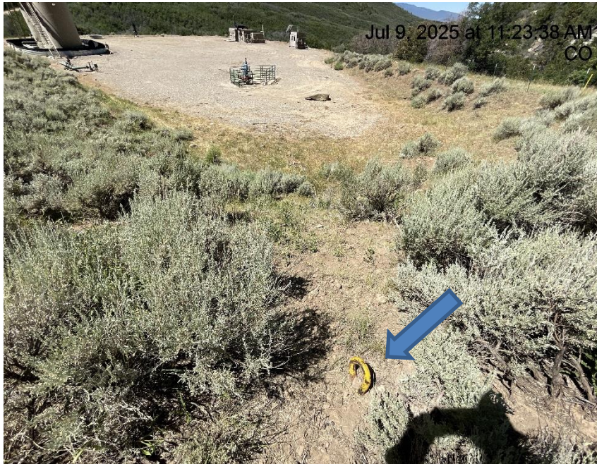
Photo # 96 Unmarked deadman
