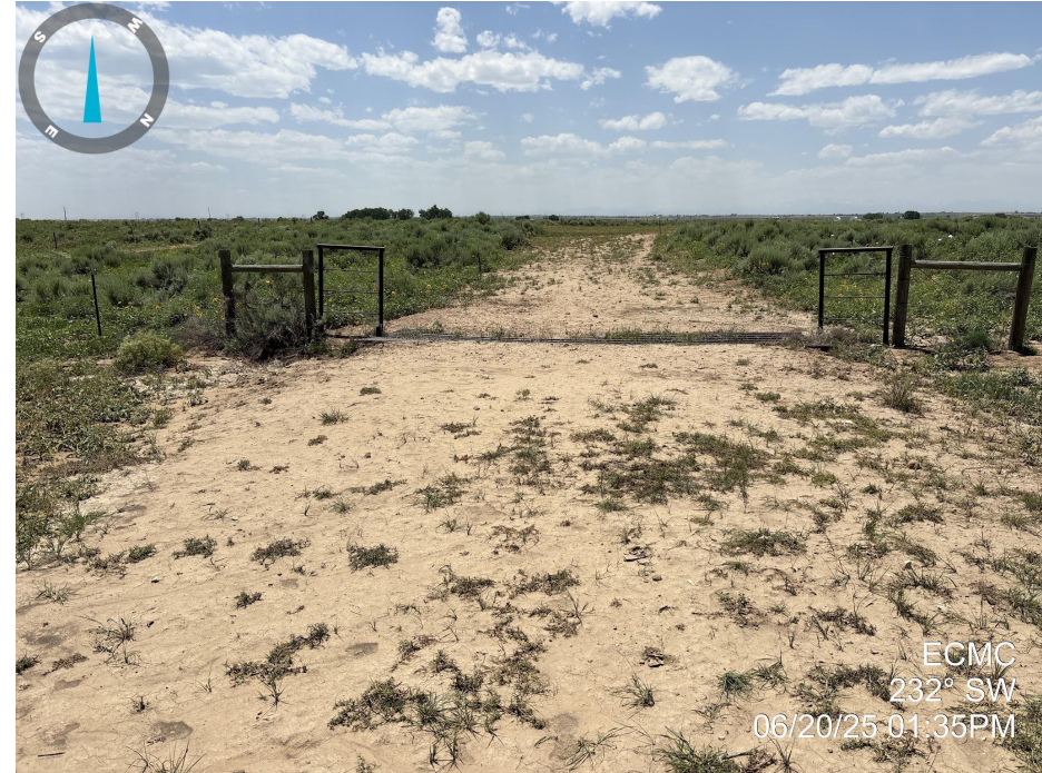
Photo 6. Photo taken of the access road, facing southwest. See comments under Photo 5.
