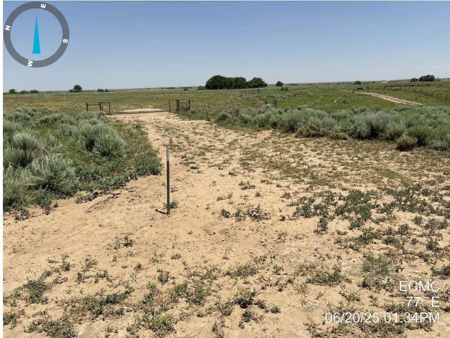
Photo 5. Photo taken of the access road to the well location, facing East. Photo illustrates that final reclamation activities have taken place, with evidence of drill row seeding, but vegetation establishment does not meet Rule 1004 standards.
