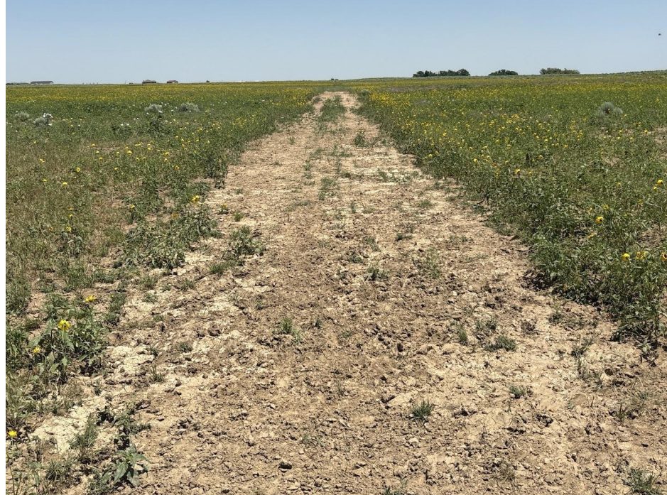
Photo 6. Photo taken of the access road, facing Northeast. Photo illustrates that final reclamation activities have taken place, with evidence of drill row seeding, but vegetation establishment does not meet Rule 1004 standards.
