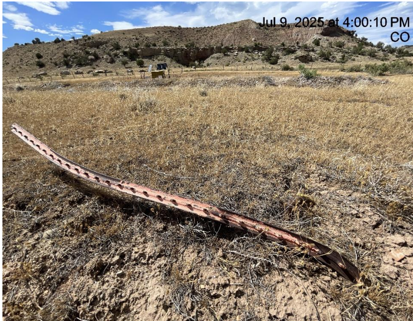
Photo # 366 Improperly marked deadman
