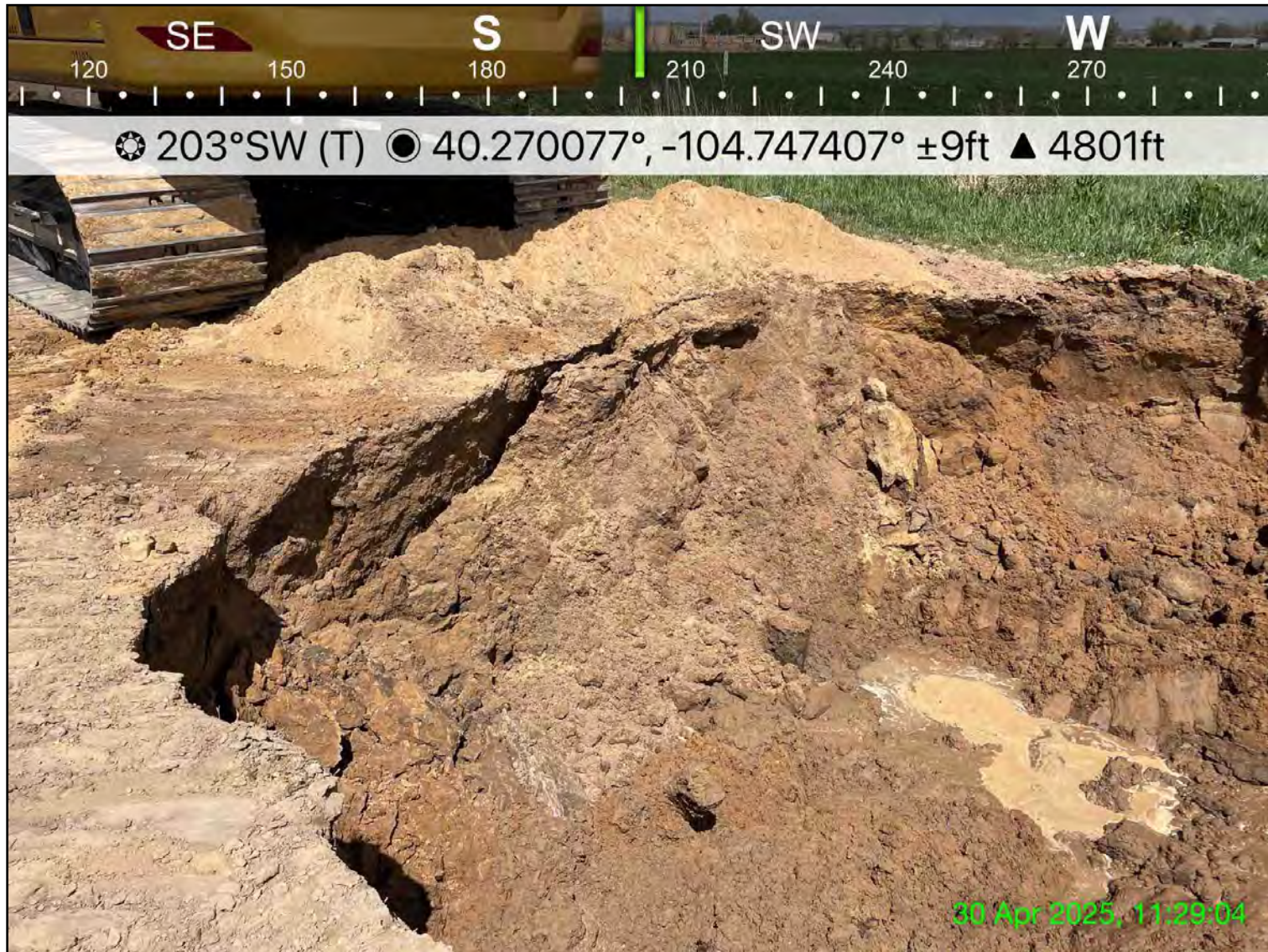
Photo 4: View of WH01-S sample location, facing southwest
