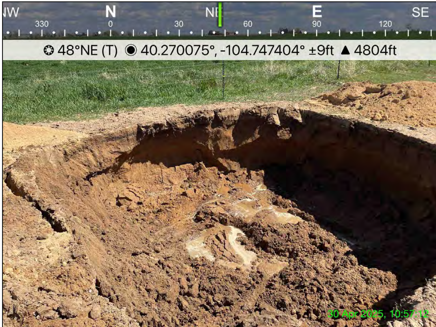
Photo 1: View of wellhead excavation filling with groundwater, facing northeast
