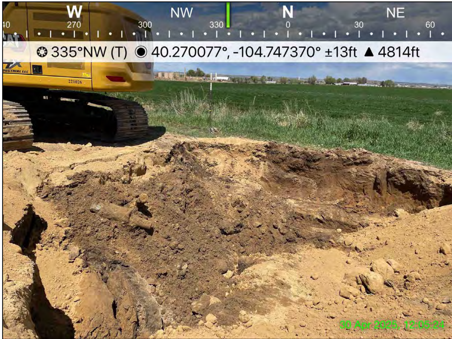
Photo 5: View of WH01-W sample location, facing northwest
