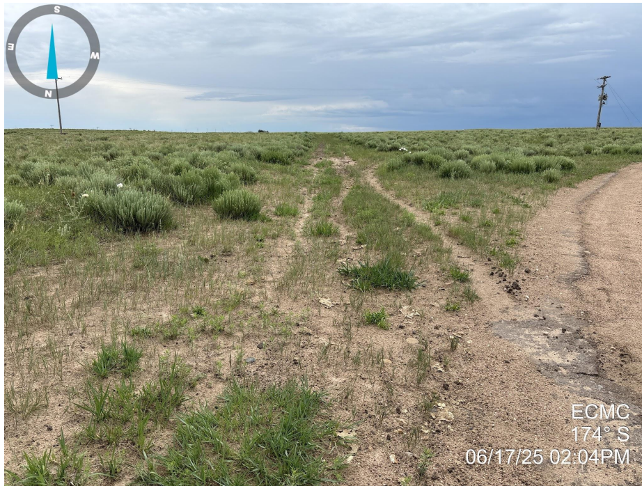
Photo 6. Photo taken of the access road, facing south towards the well location. Photo illustrates that final reclamation has not taken place along the access road.
