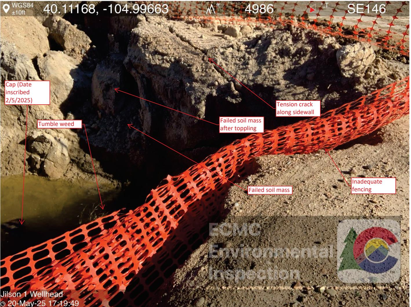
Jilson 1 Wellhead excavation - Sidewall collapse. Shallow groundwater (~5' bgs)
