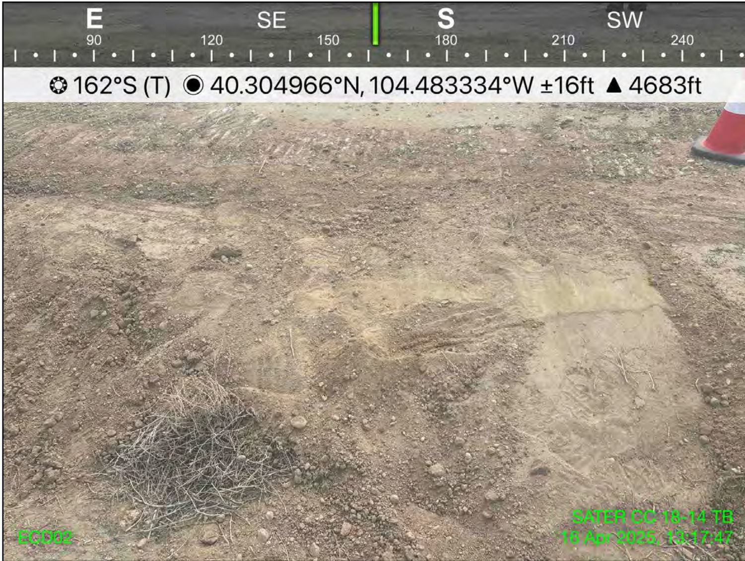
Photo 9: View of ECD02, facing south
