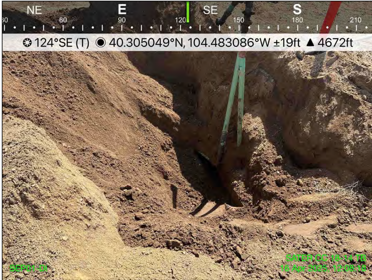
Photo 6: View of SEP01-DL, facing southeast
