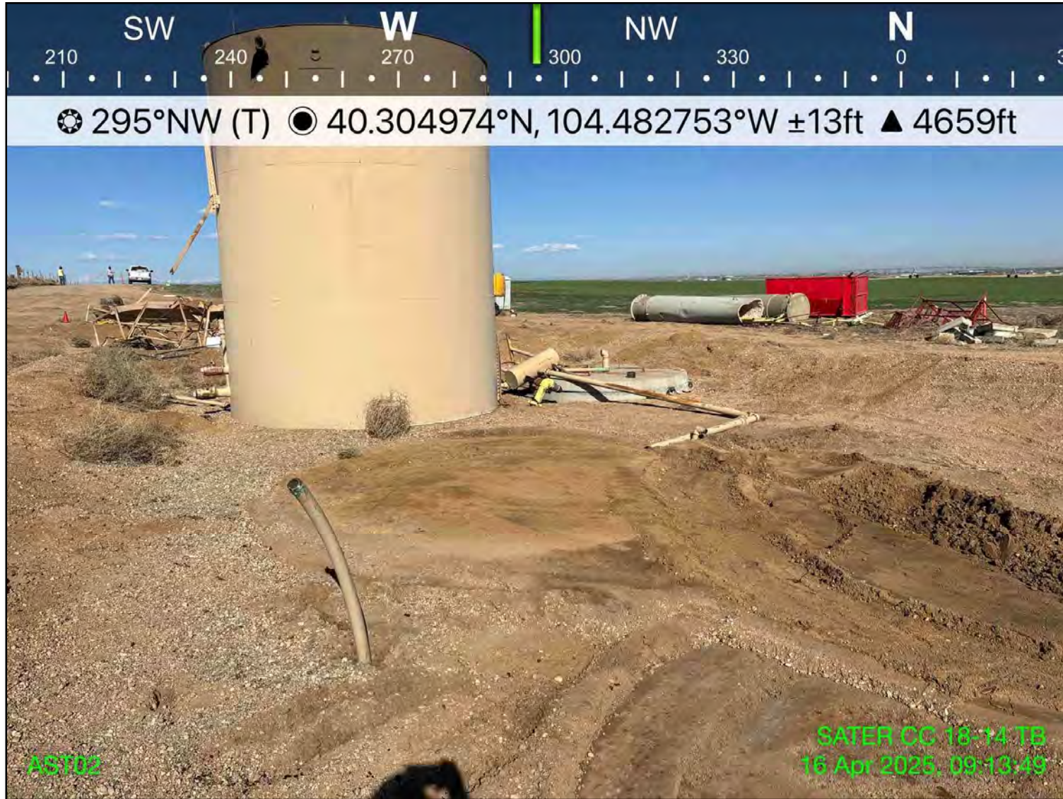
Photo 4: View of AST02, facing northwest
