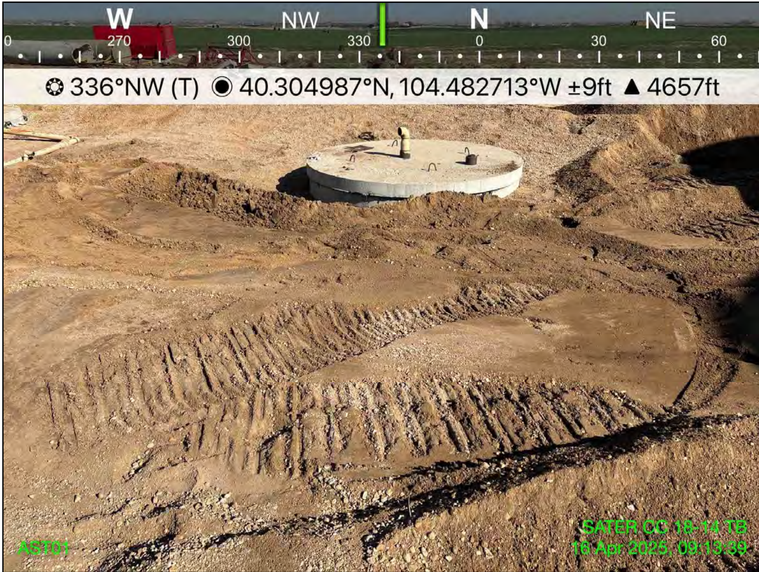
Photo 3: View of AST01, facing northwest
