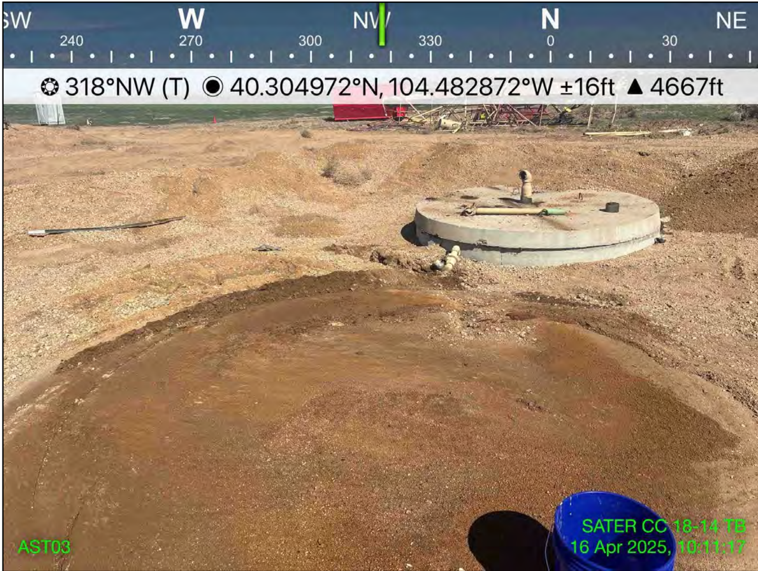
Photo 5: View of AST03, facing northwest
