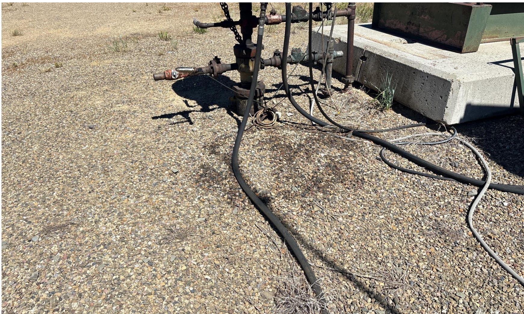
PHOTO 6: AREA OF IMPACTED SOIL NEAR WELLHEAD. Conduct maintenance on equipment, cleanup stained material and review self inspection processes. COMPLY WITH RULE 1002,(2).D. CA DATE 7-14-2025.
