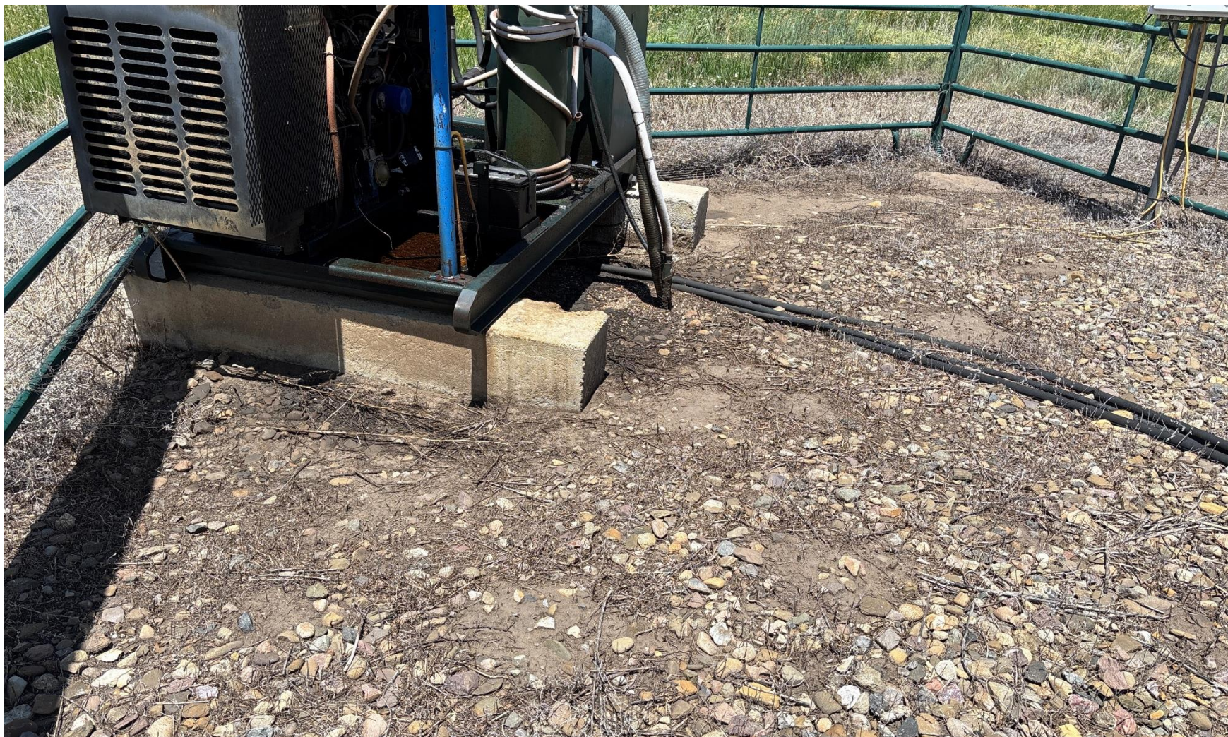
PHOTO 6: THERE IS AN AREA OF IMPACED SOILS AROUND THE PRIME MOVER ENGINE SKID. Conduct maintenance on equipment, cleanup stained material and review self inspection processes. COMPLY WITH RULE 1002,(2).D CA DATE 7-12-2025.
