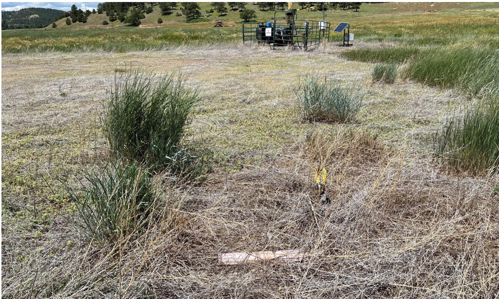
PHOTO 8: ANCHOR MARKER IS DOWN ON THE NORTH EAST ANCHOR FROM WELLHEAD. Install proper guy line markers per Rule 1003.a. CA DATE 7-2-2025 DUE TO GROWNING SEASON FARM HAND WAS CUTTING AT TIME OF INSPECTION.
