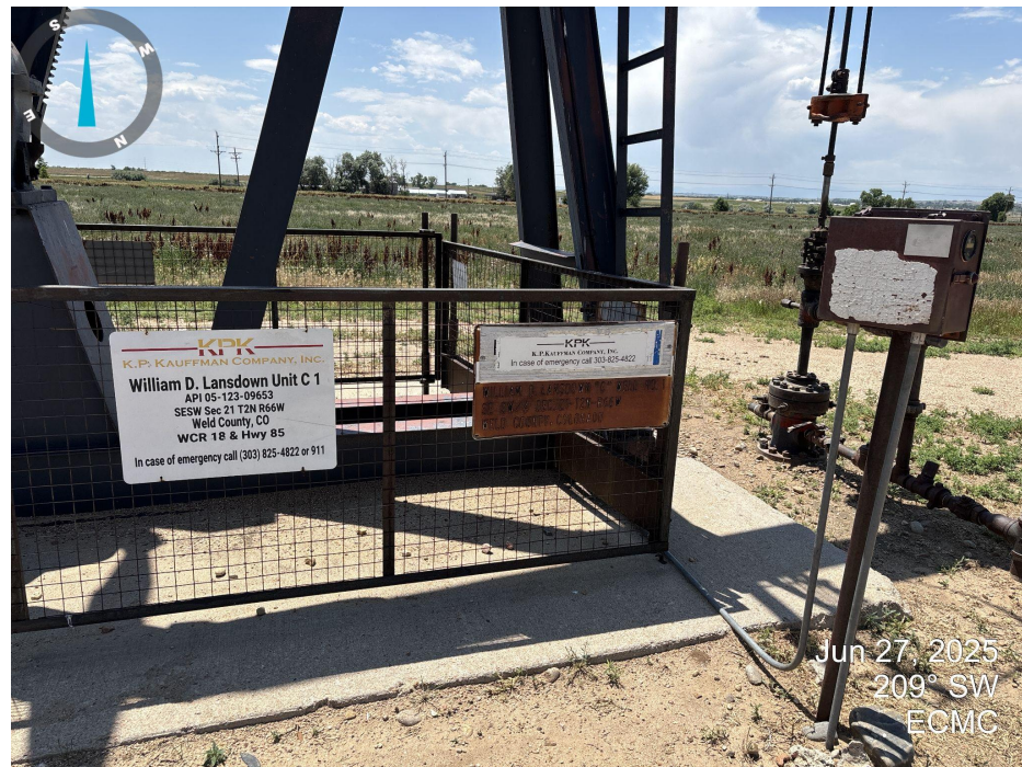
Photo 4. Looking at the north side of the pumpjack.
