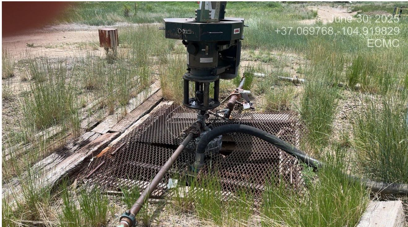
**Photo 2.** The grate does not fully cover the well cellar.
