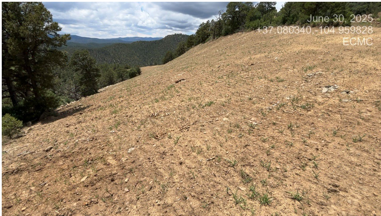
Photo 1. Facing west at the beginning of the reclaimed access road. Vegetation is beginning to emerge.
