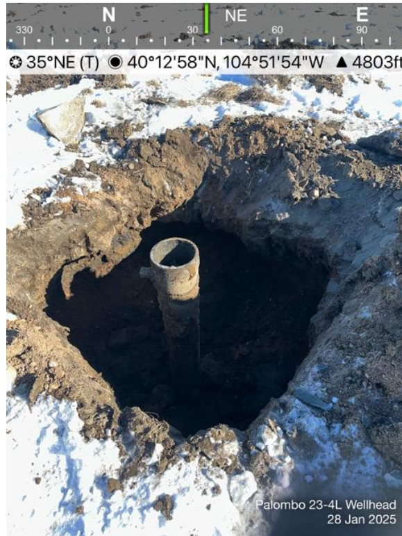
Wellhead Excavation
