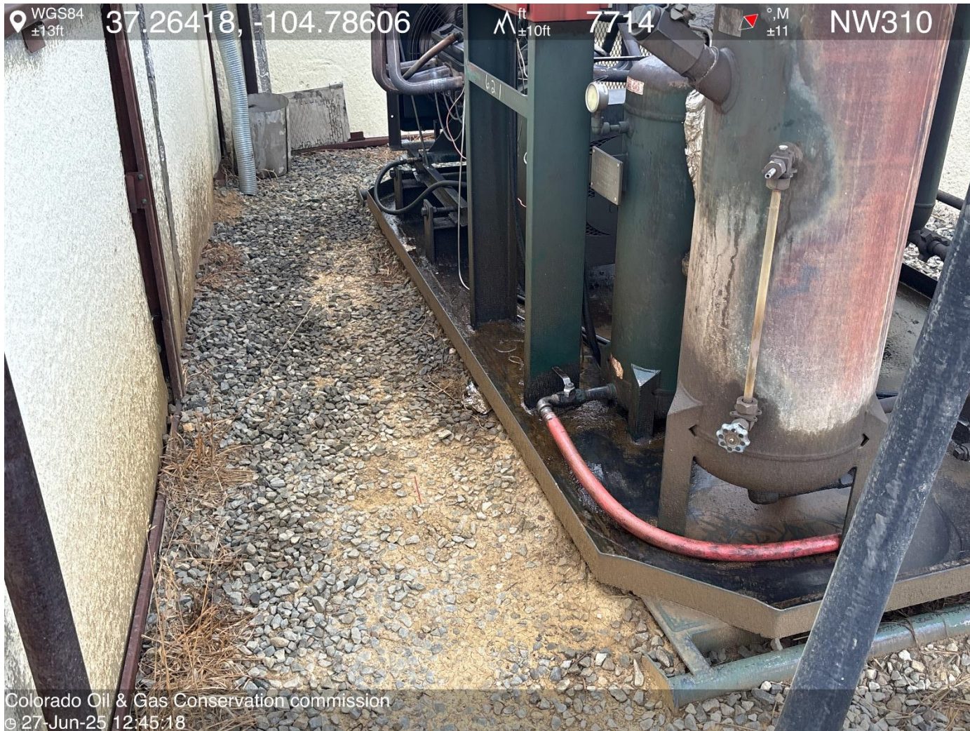
PHOTO 5: There is oil stained soil at the engine compressors and in the skids. Conduct maintenance on equipment, cleanup stained material and review self inspection processes. Conduct maintenance on equipment, FIX OR REPLACE LEAKING EQUIPMENT cleanup stained material and review self inspection processes. CA DATE 7-27-2025.
