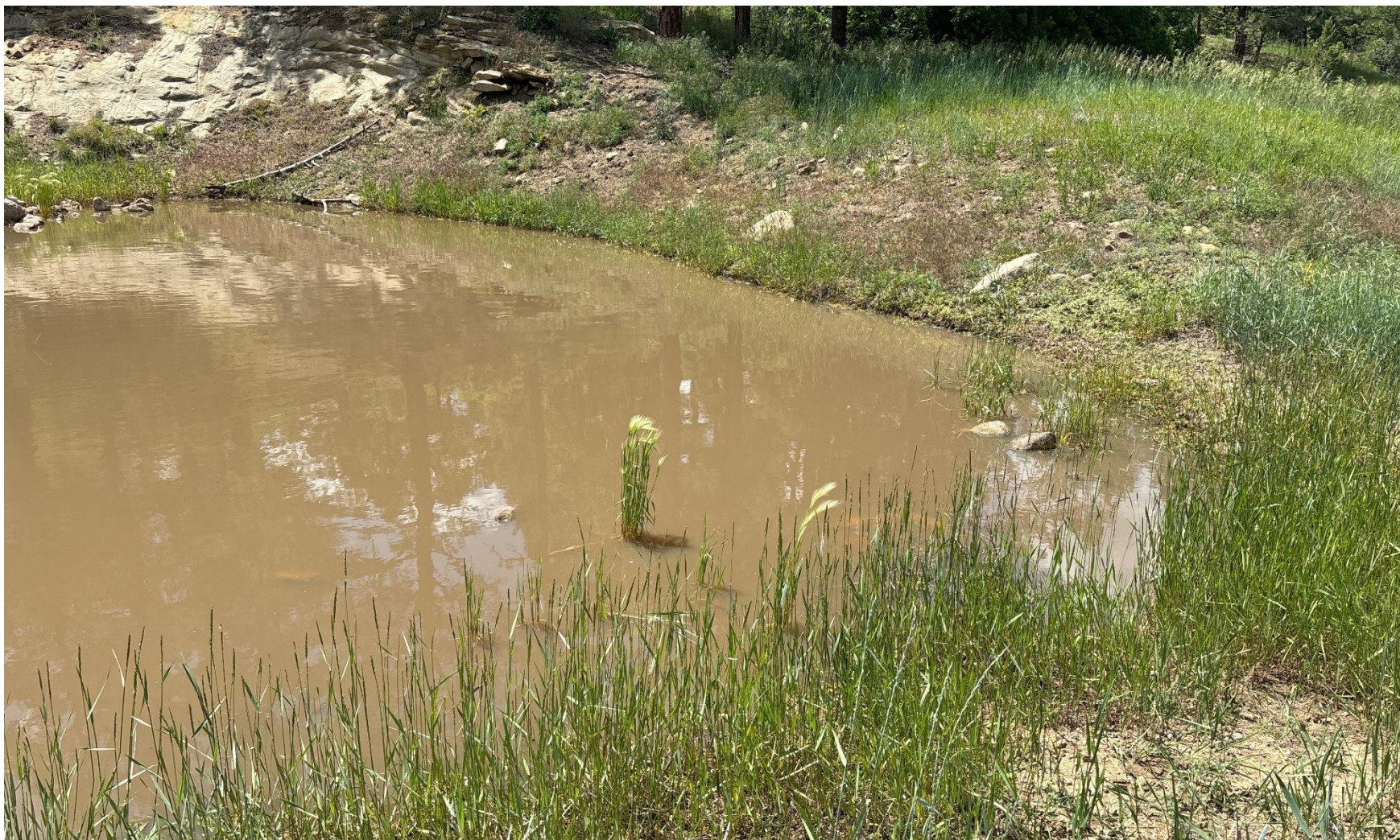
PHOTO 5: PIT LEVEL IS ABOVE FREEBOARD. Lower fluid level so at least two feet of freeboard exists per Rule 909.c. CA DATRE 6-19-2025.
