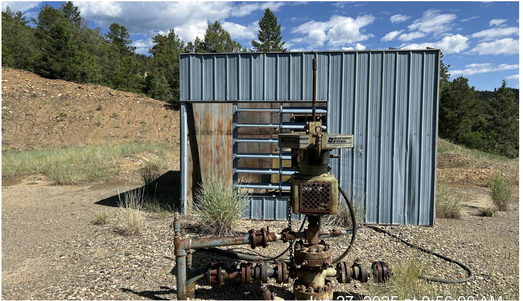
PHOTO 3: WELLHEAD AND EQUIPMENT
