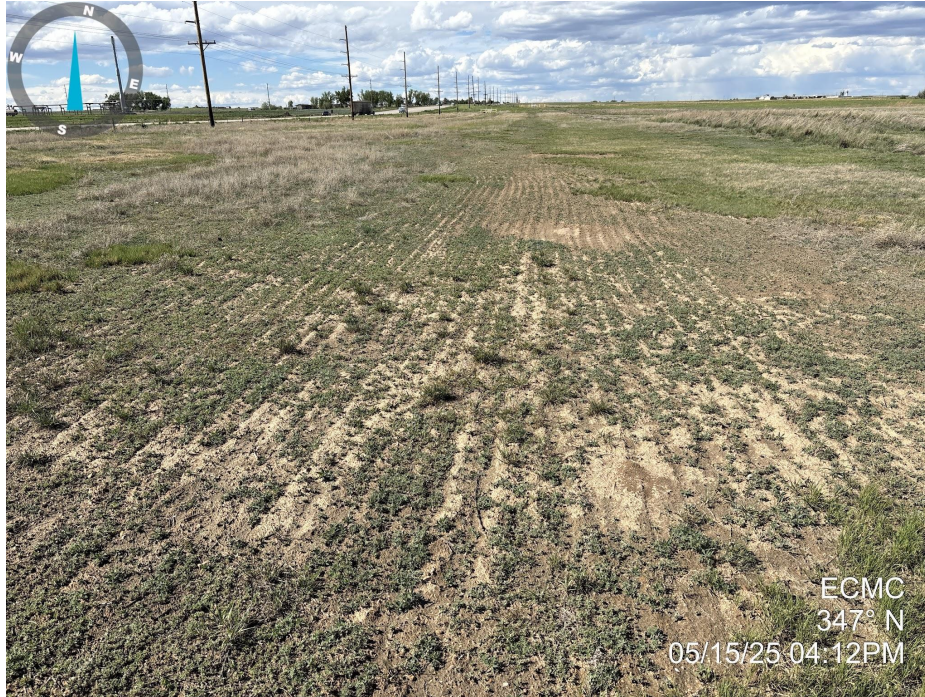
Photo 5. Photo taken from the access road, facing North towards the well location. Photo illustrates that disturbances along the access road are contained within a pipeline development following plugging of the well.
