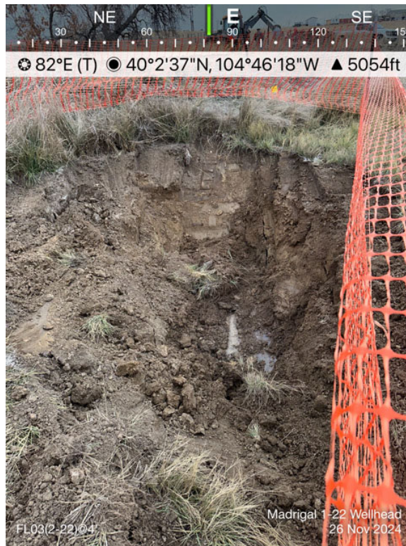
Flowline Sample Location 03
