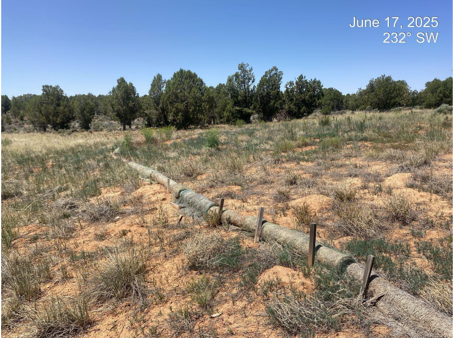
Photo 3. Wattles with plastic wrap remain on location.
