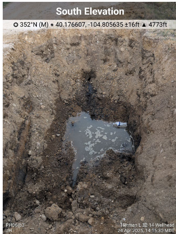
PH06 Screening Location (Groundwater Present)
