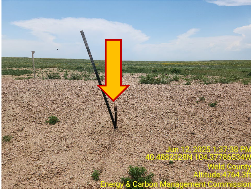
Photo 5 – Unmarked Riser
