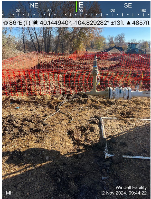
Meter House Screening Location
