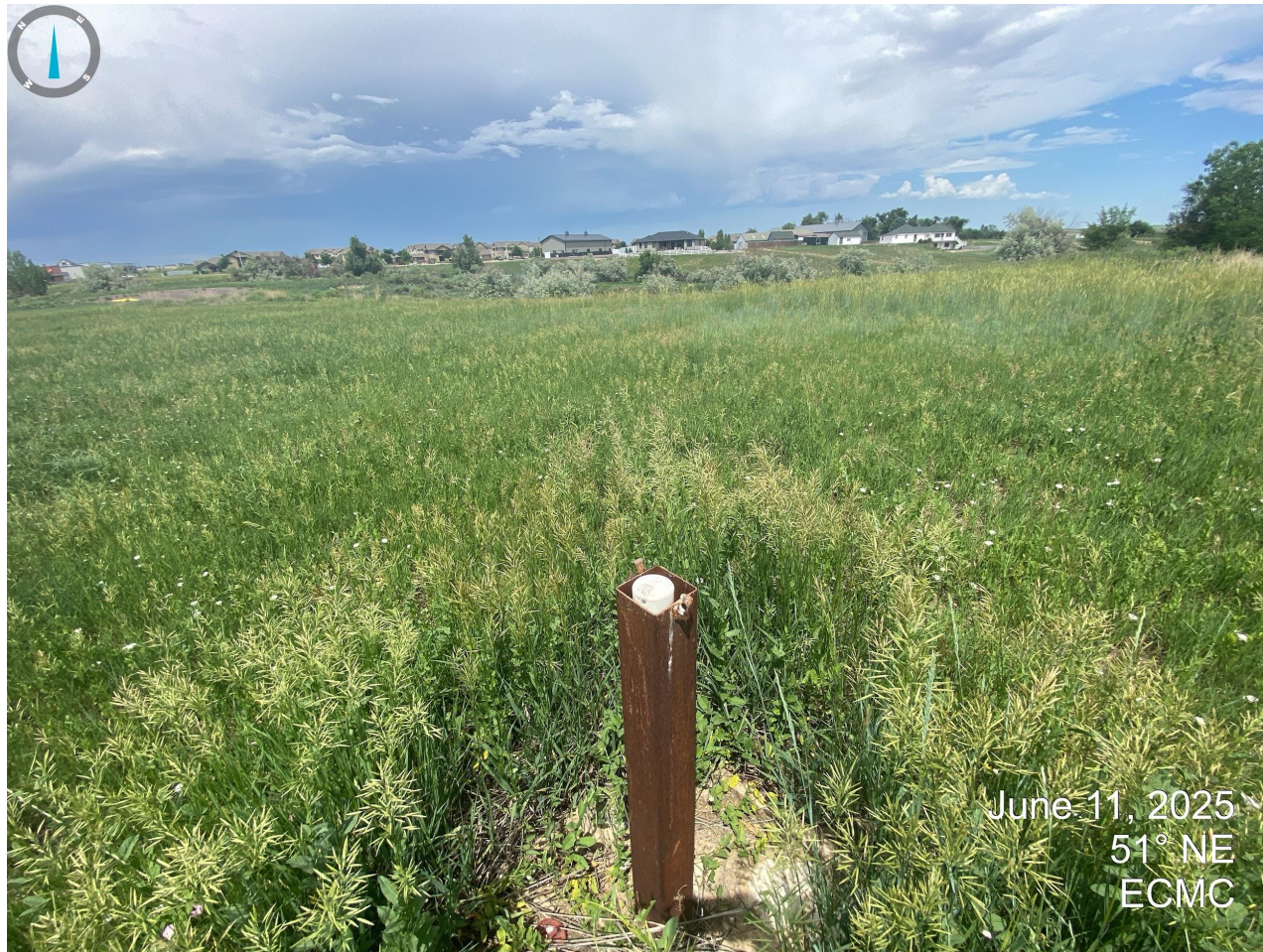
Photo 11. Continued from Photos 9 & 10. Groundwater monitoring wells remain around the former well location and will need to be removed.
