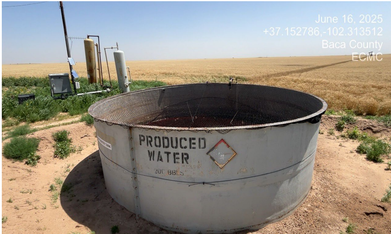
Photo 2. The netting on the tank has been repaired and maintained.
