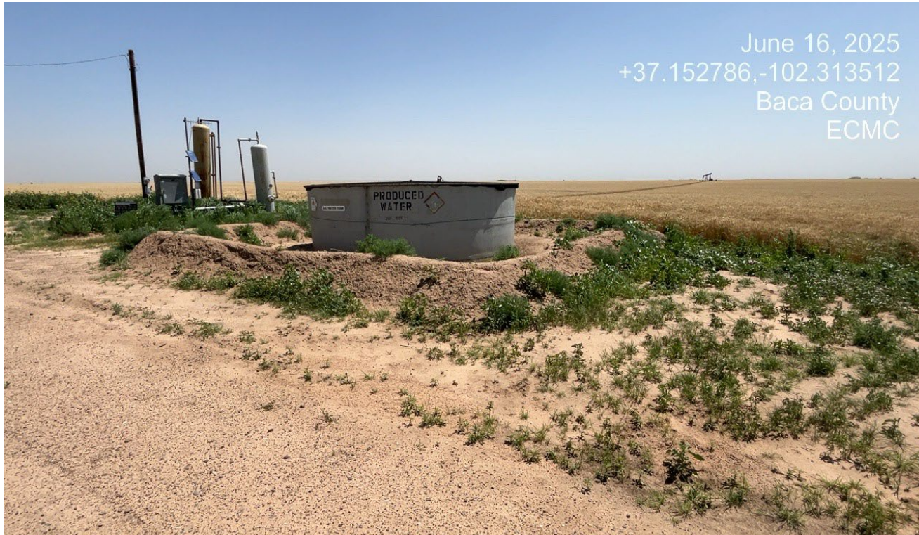
Photo 1. Facing northeast toward the offsite tank battery. The tank berm has been rebuilt for sufficient secondary containment.
