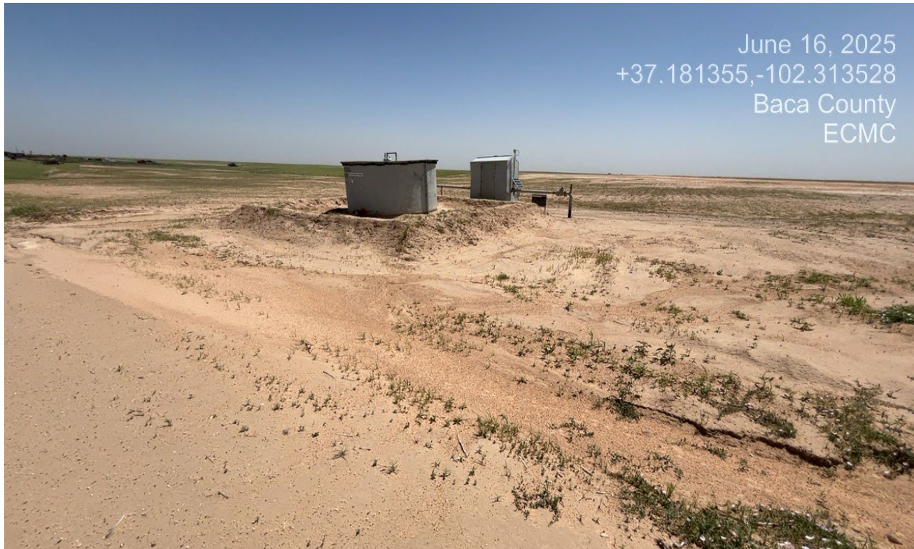
Photo 1. Facing north toward the offsite tank battery. The tank berm has been rebuilt for sufficient secondary containment.
