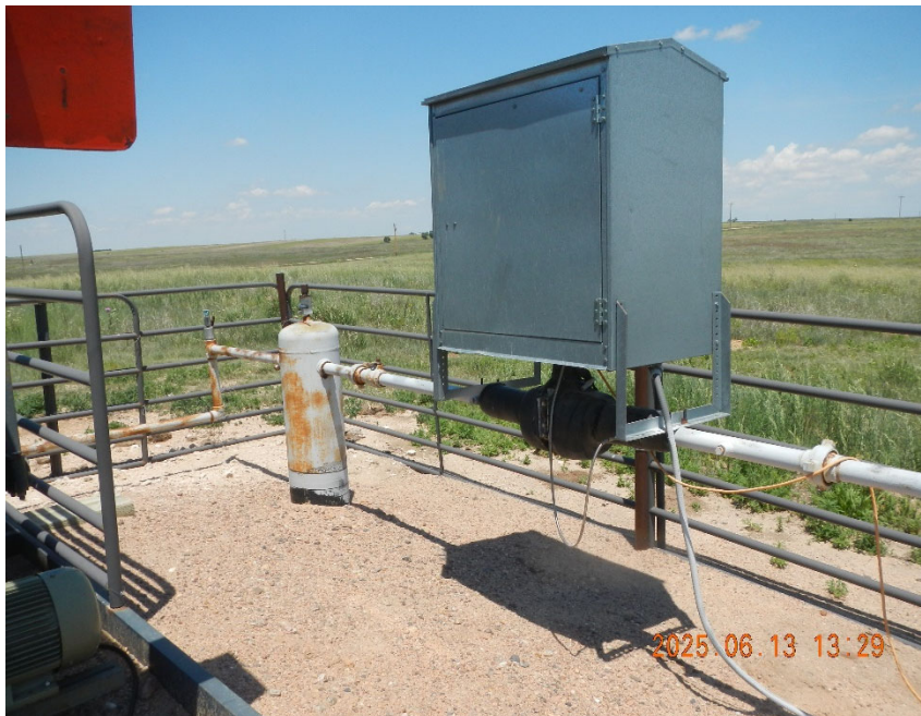
3. View of Meter Box and Dehydrator inside well fencing.
