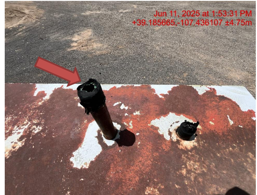
Photo # 8371 PRV vent line does not comply with CECMC pressure safety device rules
