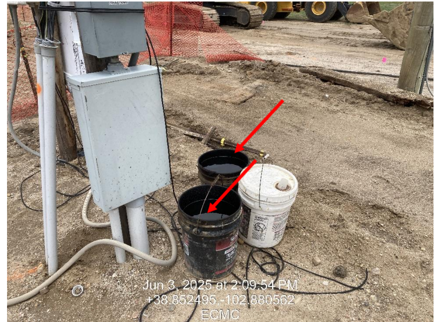
Photo 6 – 5 gallon buckets with no containment
