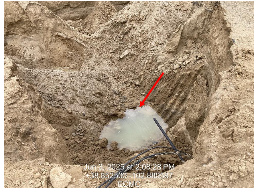
Photo 4 – Groundwater in excavation
