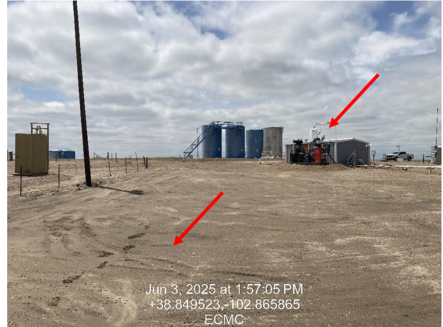
Photo 6 – Spill area and new compressor.
