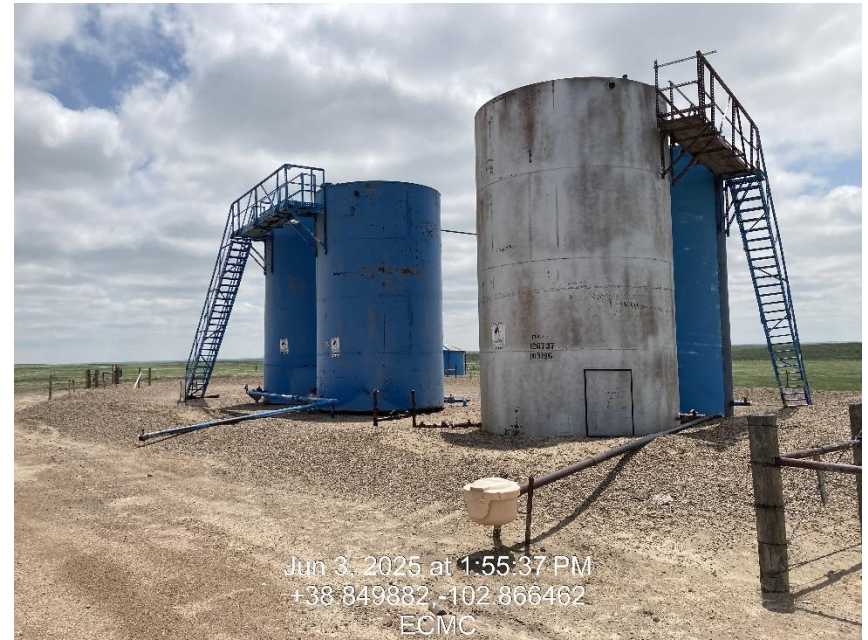
Photo 2 – Tank battery
