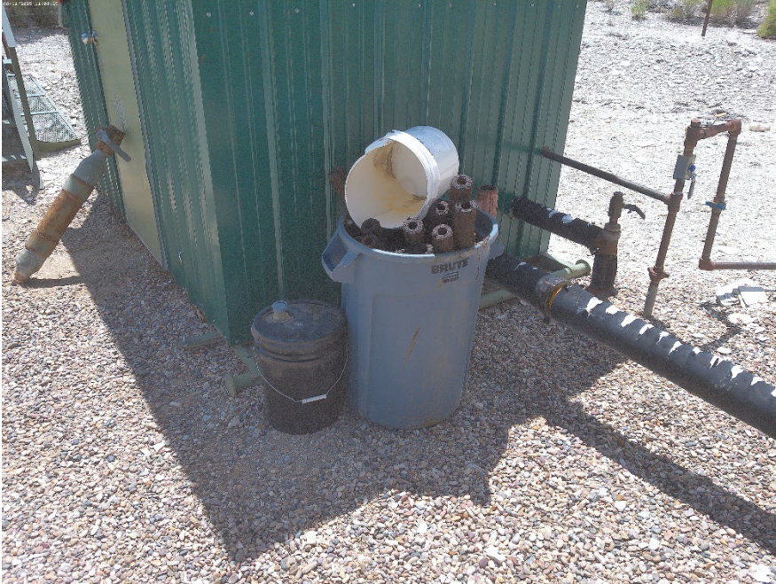
Used filters socks outside pump housing
