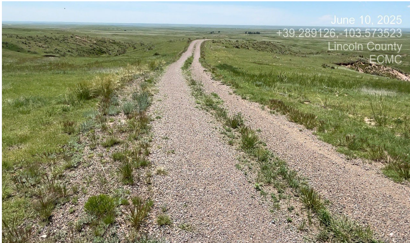
Photo 1. Facing south along the access road. Gravel along the road will need to be removed and the road will need to be reclaimed.
