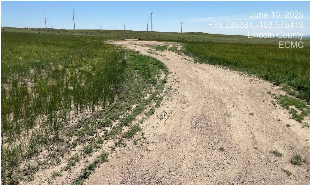
Photo 3. Facing southeast at the location. The location has not been recontoured and reclaimed.
