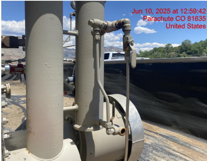
PRV Terminates in Unsafe Manner – Photo #09234
