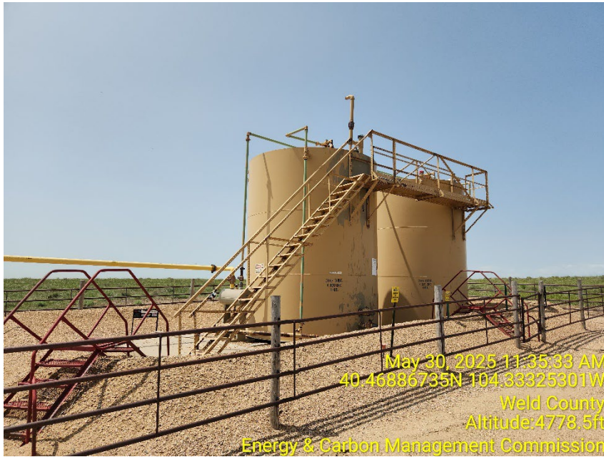
Photo 1 – Tank Battery
