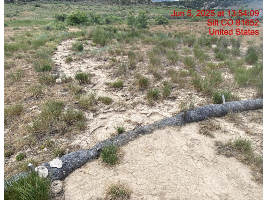
BMP Failure/Transport of Sediment Offsite – Photo #09170
