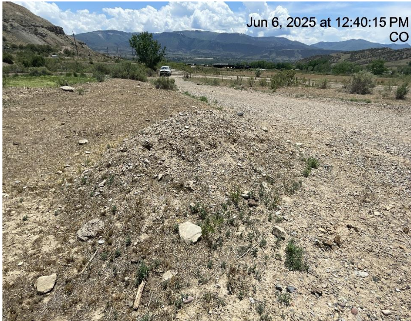
Photo # 7709 Soil stockpile with no BMP's
