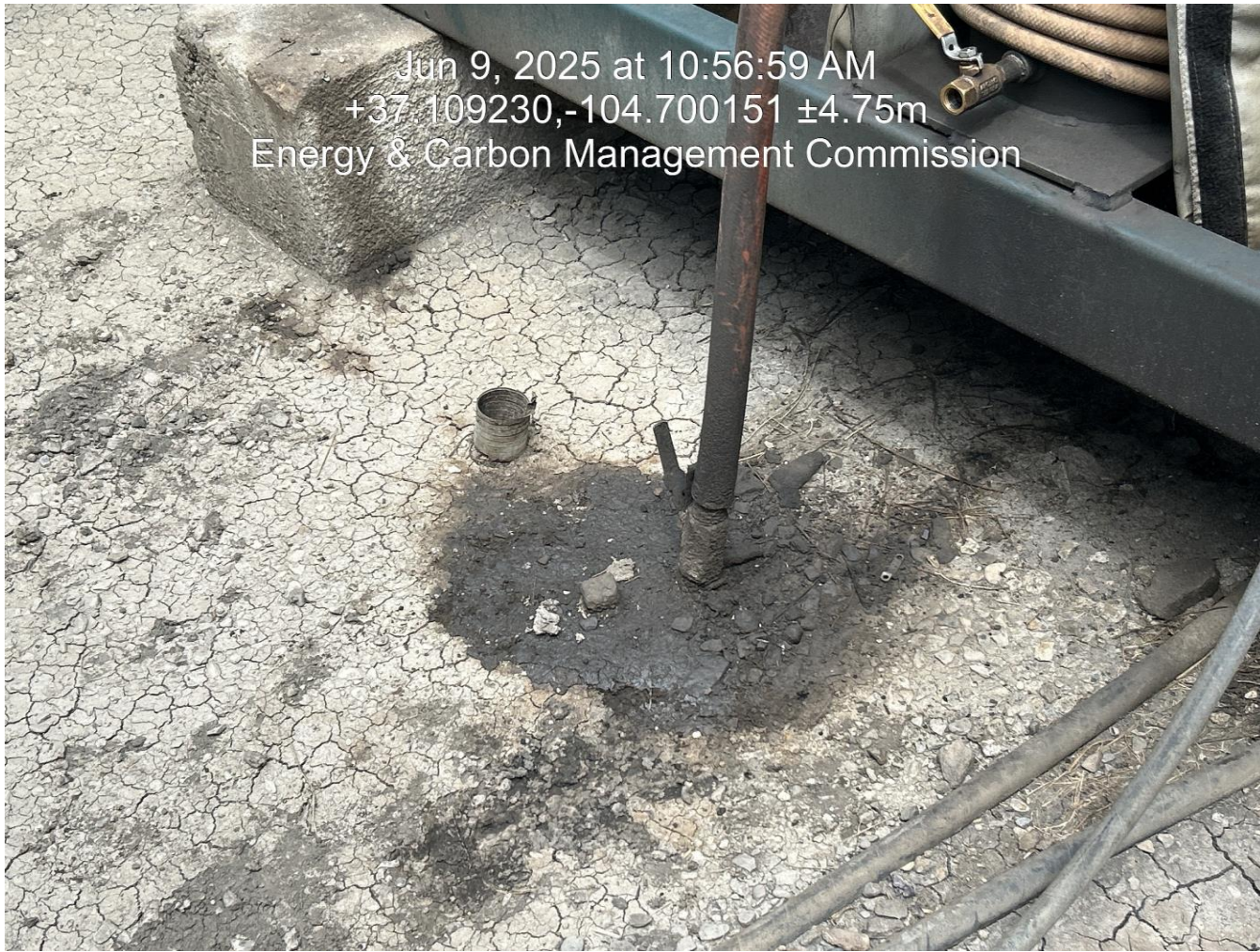
PHOTO 5: Stained soil around engine skid
