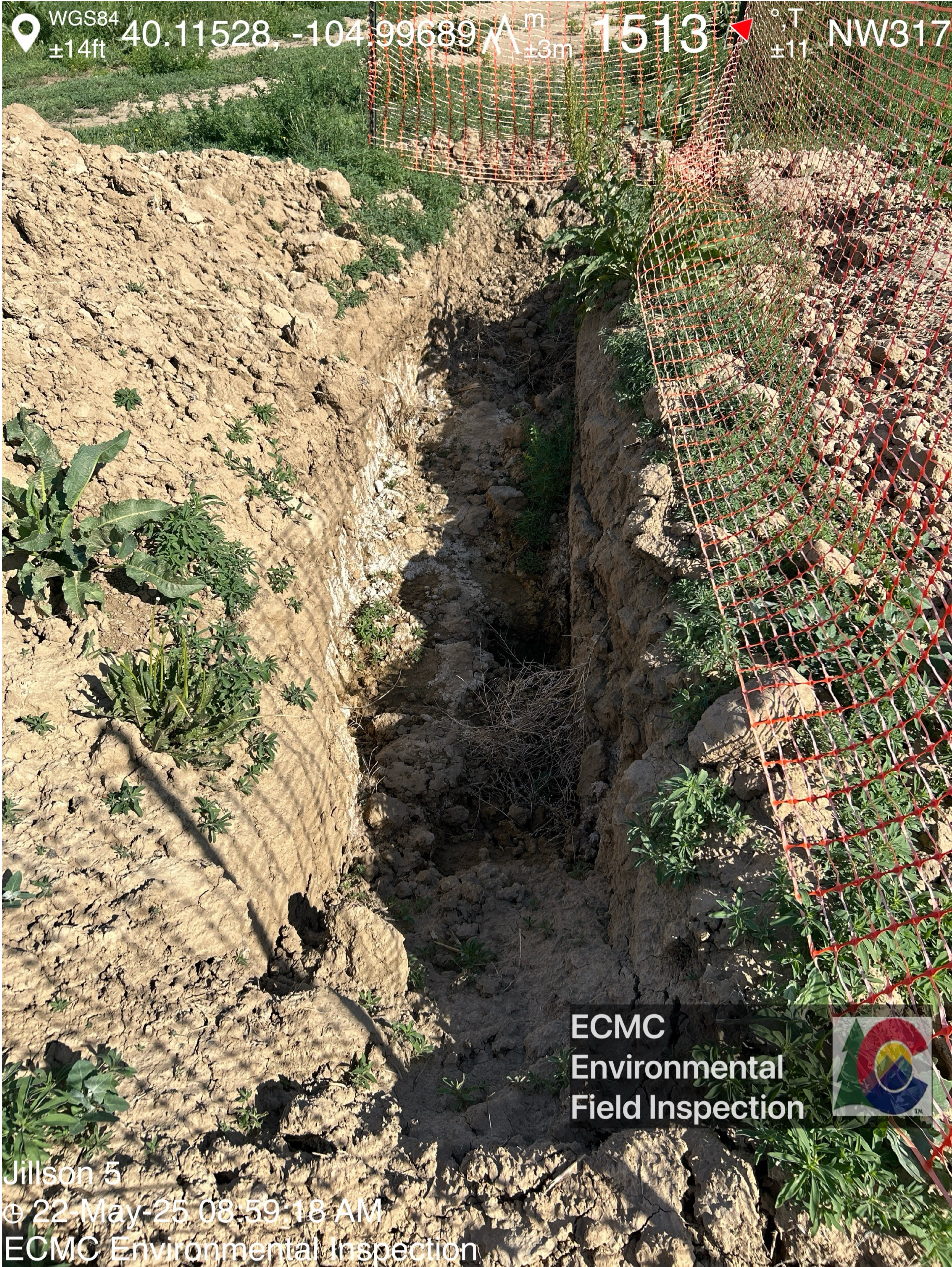
Salt crusting was visible within the southeastern trench. Orange construction fencing and plastic tape partially surrounds the trench but does not fully encompass the perimeter.
