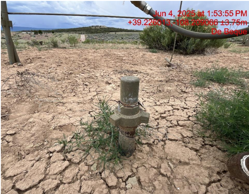
Photo # 7716 Intermediate Casing valve is buried/not in compliance with CECMC rules
