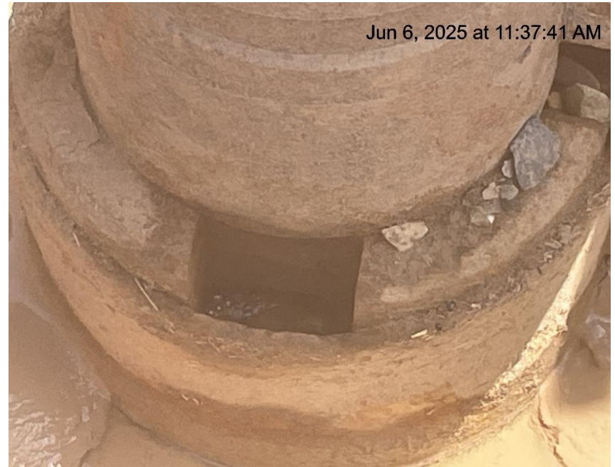
Photo # 7213 UNOCAL-ENCANA 14A-9D wellhead leak
