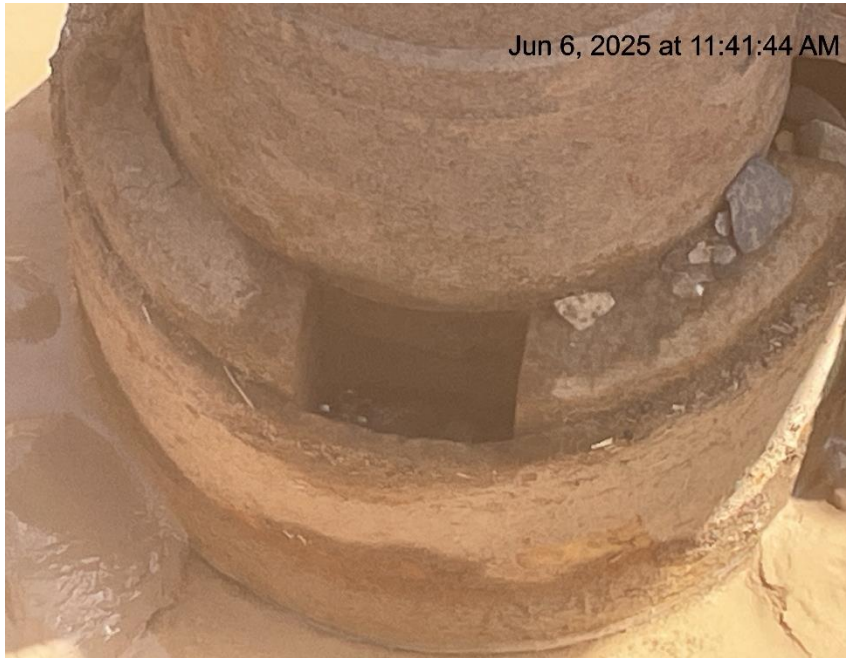
Photo # 7212 UNOCAL-ENCANA 14A-9D wellhead leak
