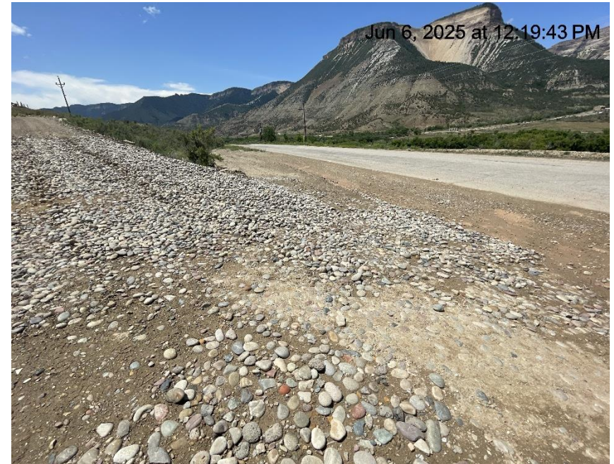
Photo # 7238 Tracking pad/BMP at intersection of CR 215 & start of lease road has not been improved
