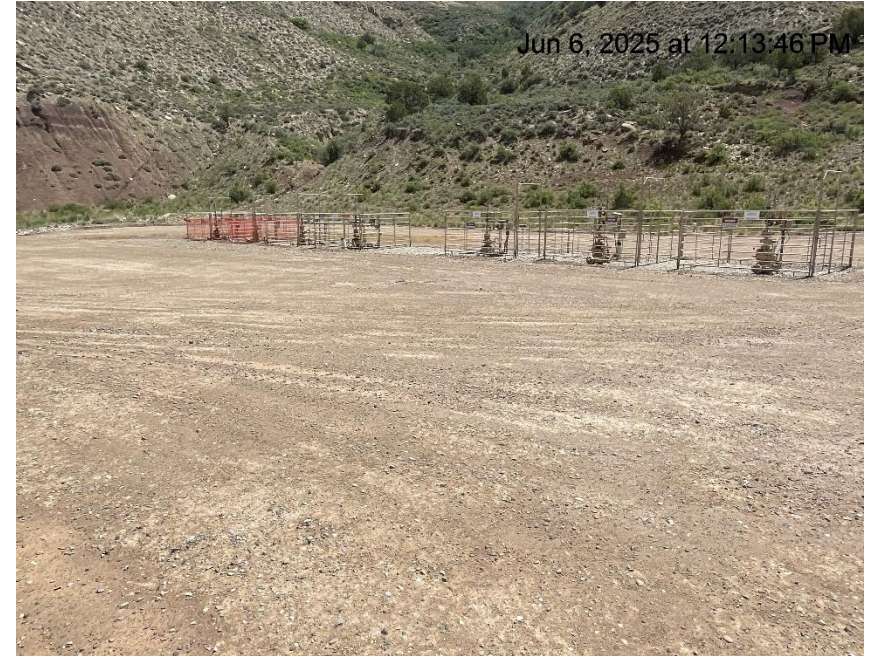
Photo # 7232 BMP's have not been added to stabilize the working surface of the pad
