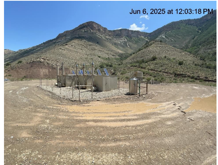
Photo # 7230 BMP's have not been added to stabilize the working surface of the pad
