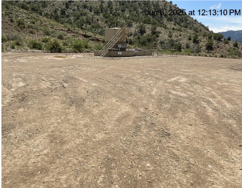
Photo # 7231 BMP's have not been added to stabilize the working surface of the pad
