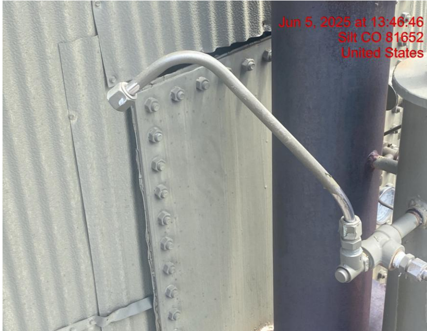
PRV Terminates in Unsafe Manner – Photo #09159
