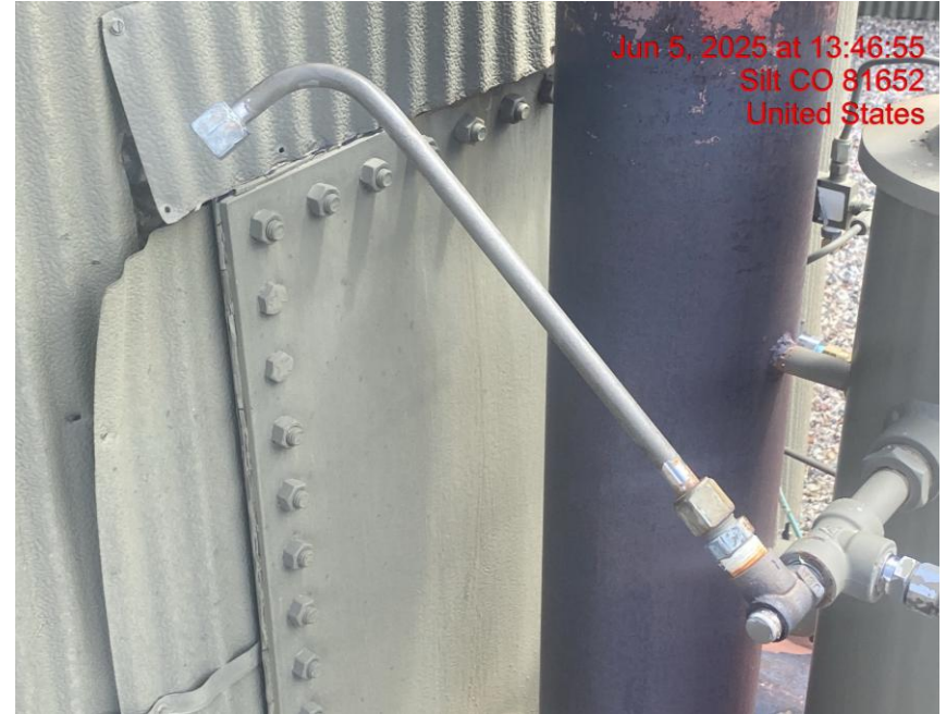
PRV Terminates in Unsafe Manner – Photo #09160
