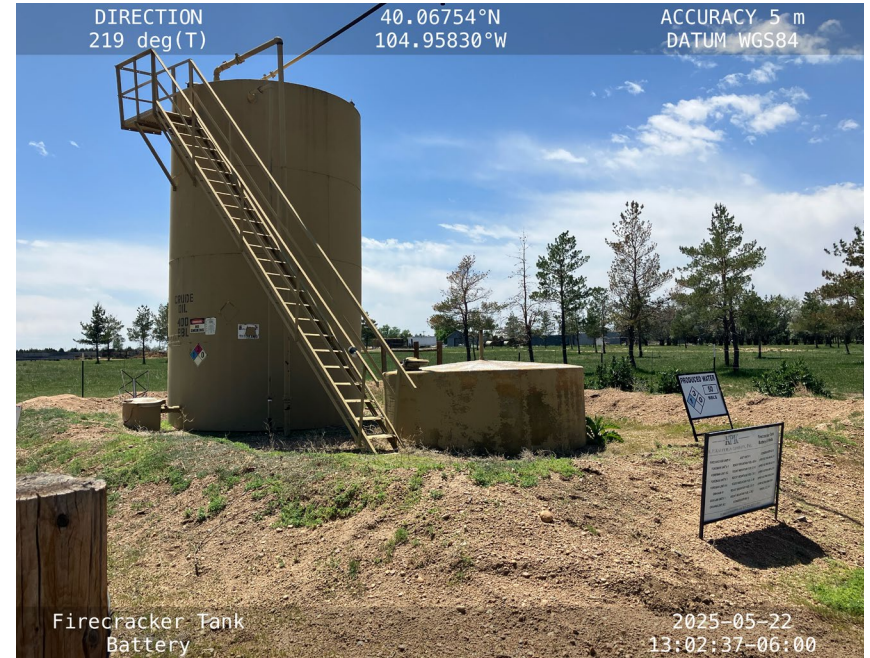
Weeds and inadequate earthen berm
