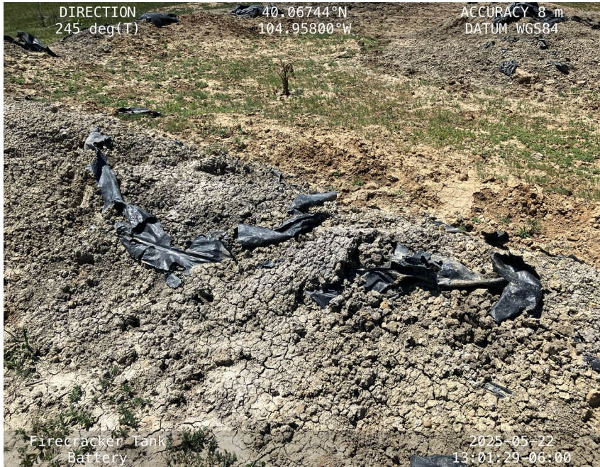
Oily waste within stockpile. Torn liner
