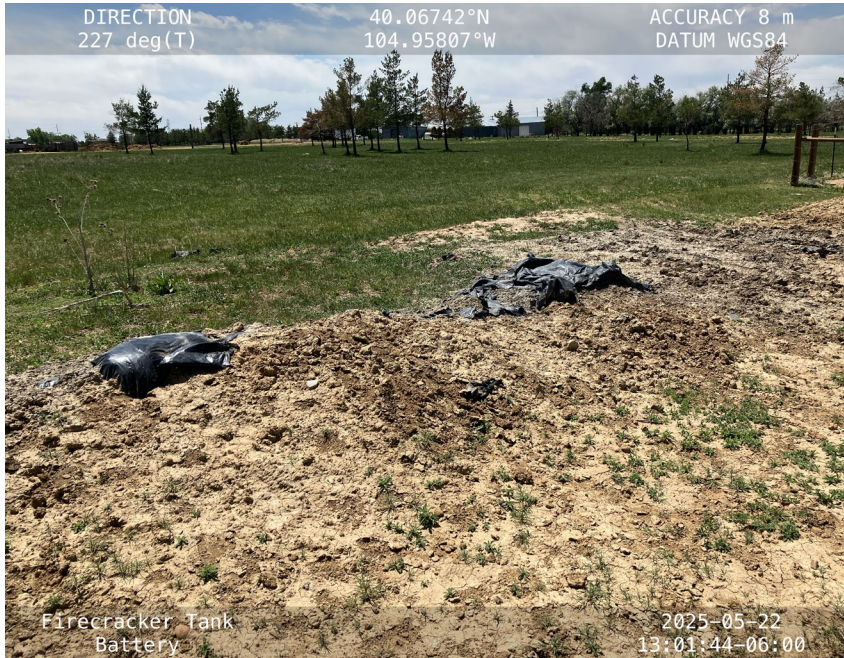
Oily waste within stockpile. Torn liner
