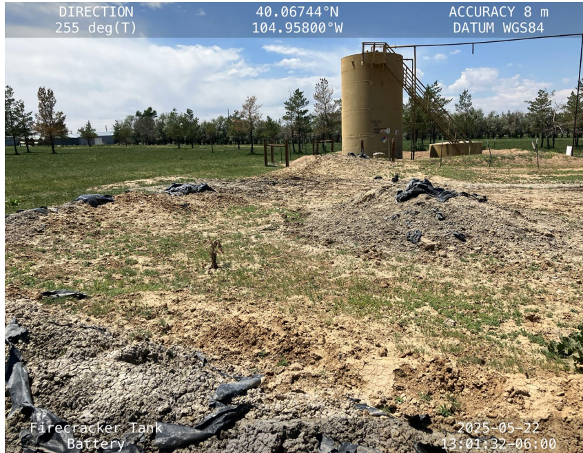
Oily waste within stockpile. Torn liner
