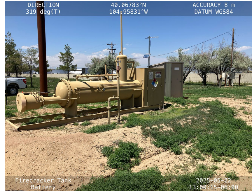
Weeds and inadequate earthen berm
