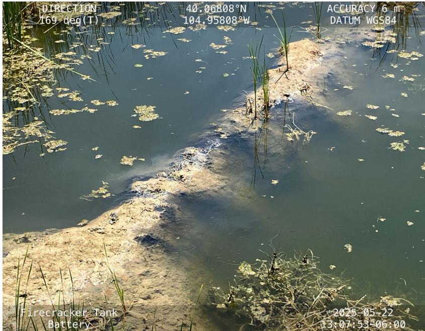
Excavation with groundwater. Oil-stained soil along the flowline
