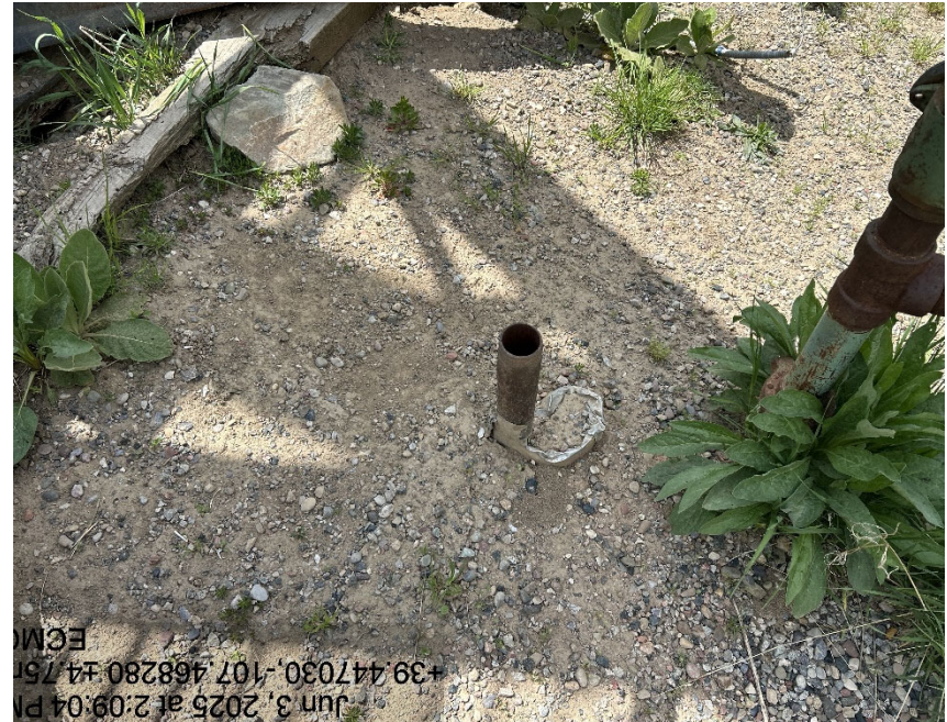
Recent inspection C/A still present
